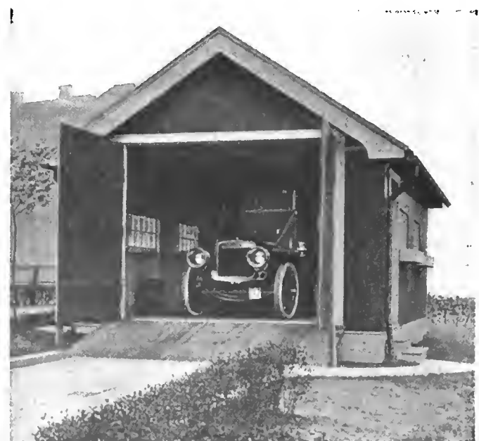
Front View and Exterior of Small Portable Garage Above
